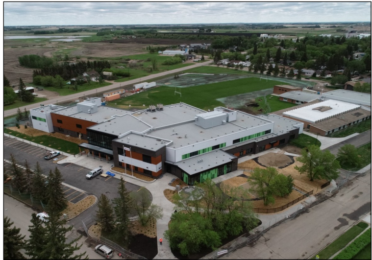
Drone view of Rosthern Community School, June 2020 (Rosthern High School is on the far right with the white/brown roof)
